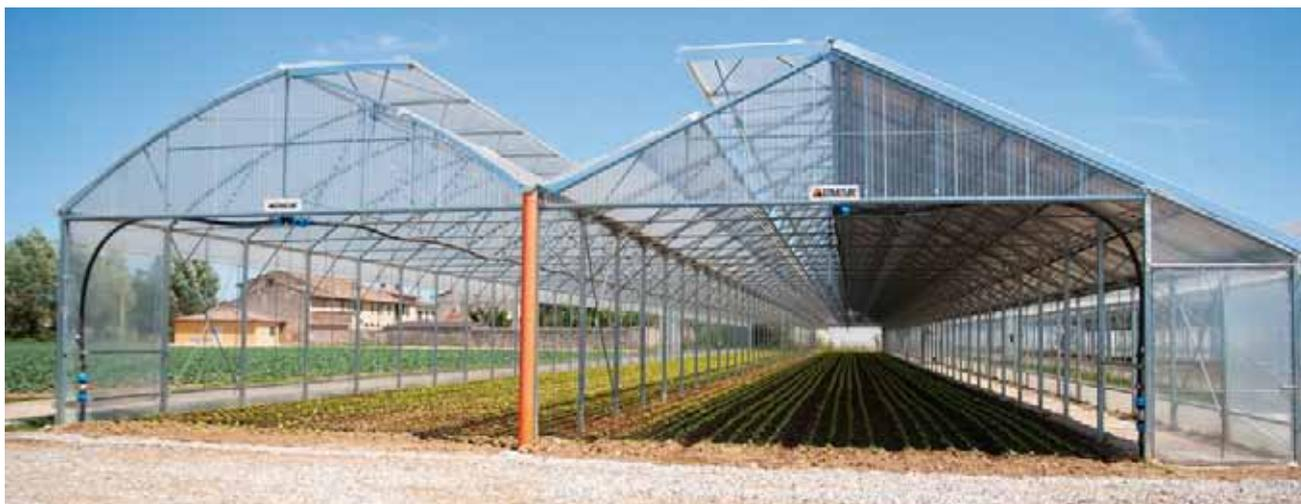
Each plant is dimensioned to support the wind and the snow overloads, accordingly to the specific site conditions where it is installed. For each plant, we present the 10 years Guarantee Certificate and the declaration of entire system disposal at the life end.
